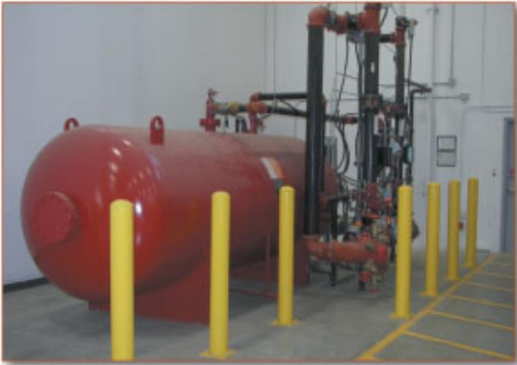
**JD's** distribution center utilizes innovative equipment for safety, such as this tank of foam to suppress a fire from spreading.
