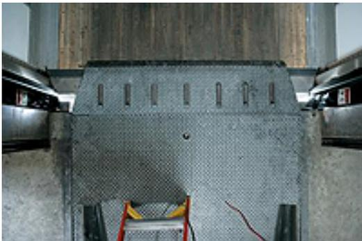
**A common example** of dock leveler gaps that can be a major cause of energy loss and unnecessary cost.
